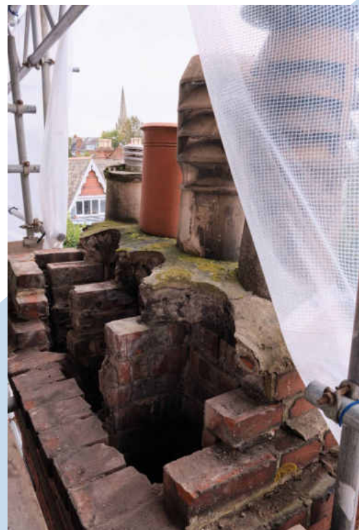
The wall of the damaged chimney was bowed and needed rebuilding.
