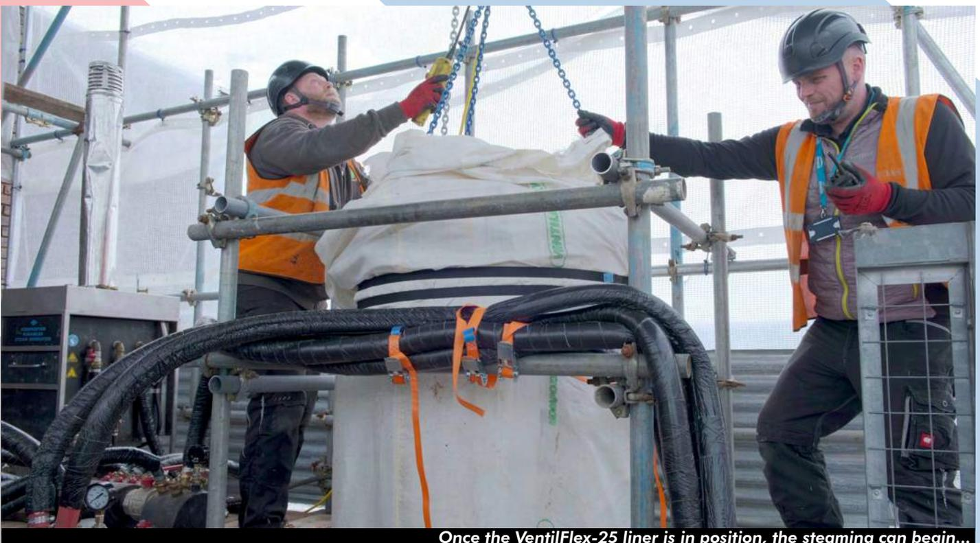
Once the VentilFlex-25 liner is in position, the steaming can begin...
