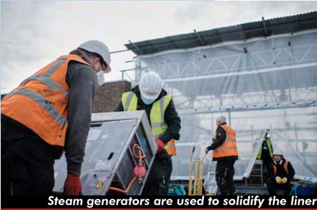
Steam generators are used to solidify the liner
