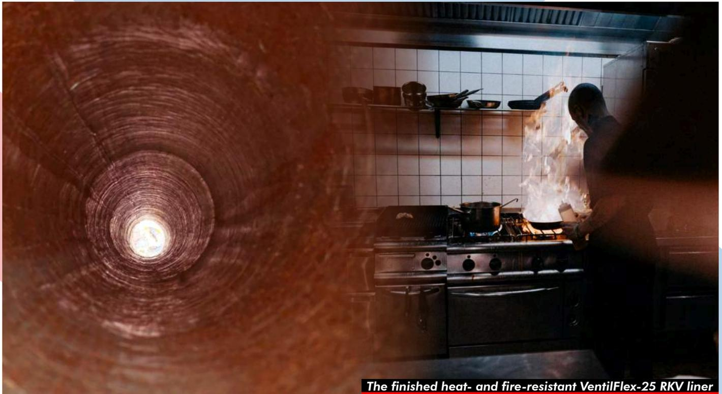
*The finished heat- and fire-resistant VentilFlex-25 RKV liner*
