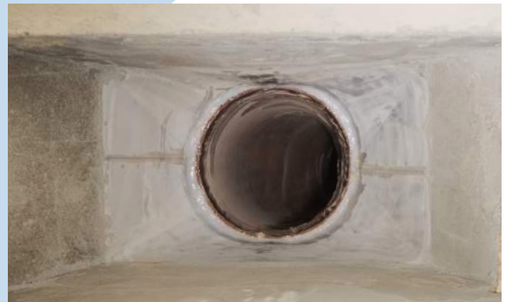
The finished flue.
