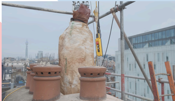
VentilFlex-25 liner during steaming.
