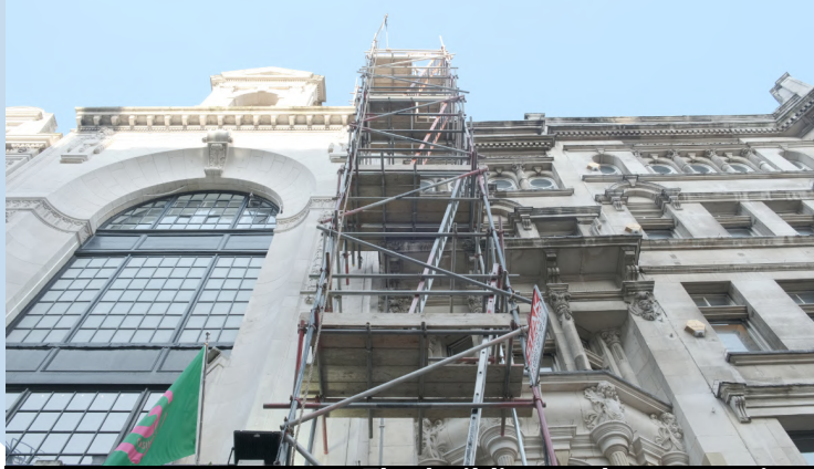
The building under renovation.
